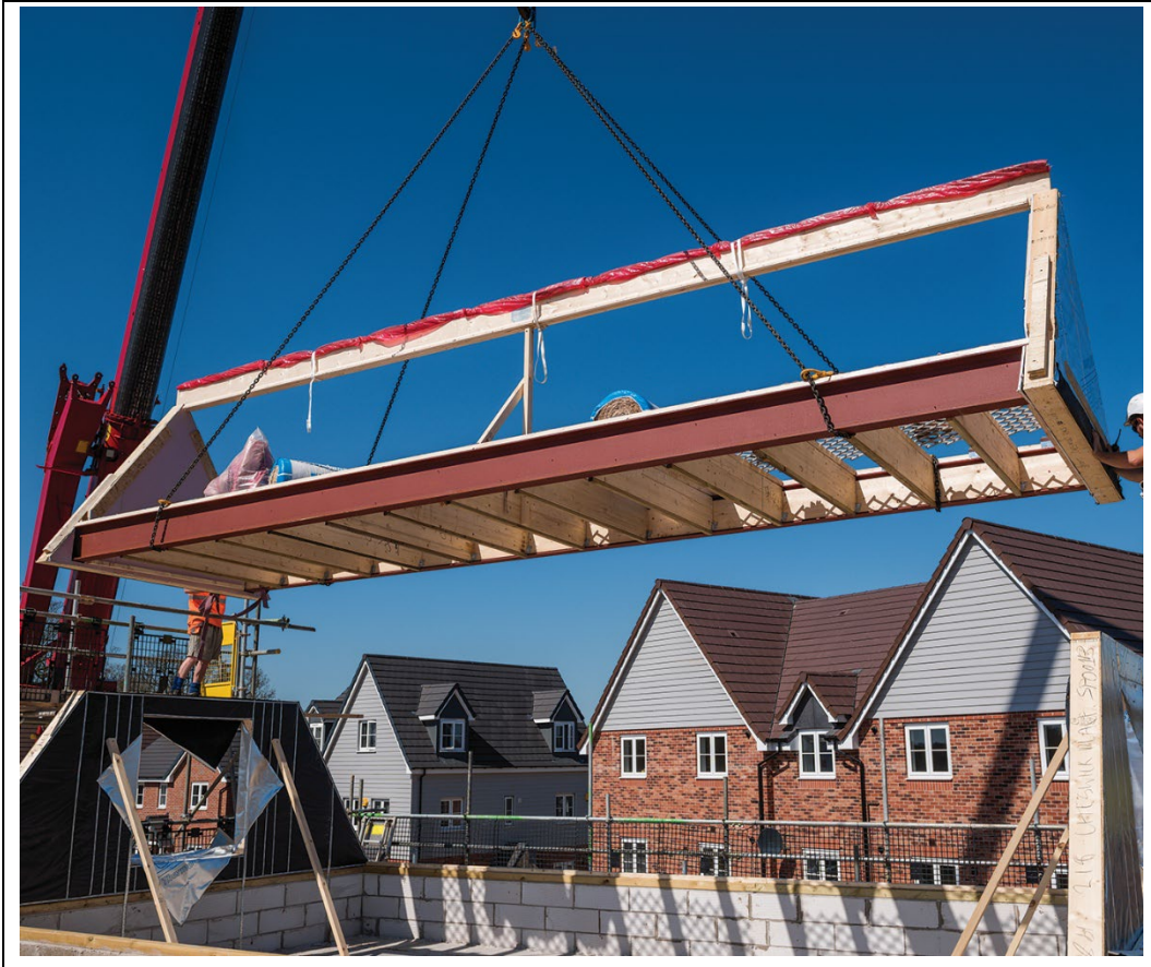
Figure 5 Top hat assembly being lifted into place
