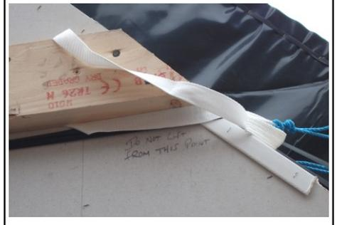
4. Once the order of unloading is agreed between the slinger and driver the slinger will attach the purple lifting slings to the crane hooks.
