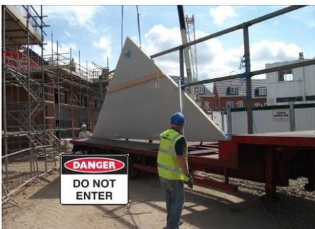
9. Repeat the process for the remainder of the panels. Small clad panels will be secured to a pallet with heavy duty strapping and purple lifting slings attached for ease of off-loading.
