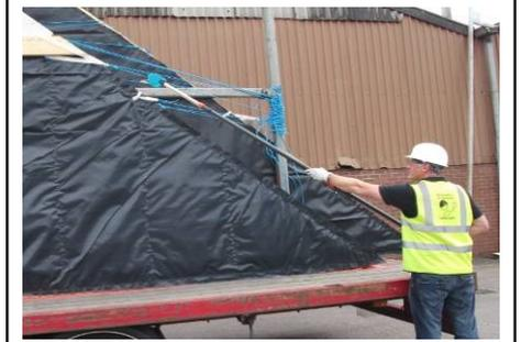
8. The crane will lift the panel from the bed of the trailer. **NEVER** stand in the danger area where the lifted panel could
