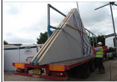
6. On instruction from the site responsible person the driver will cut the blue rope which attaches the individual panel to the centre bar using the cutting device, and standing outside of the danger area.
