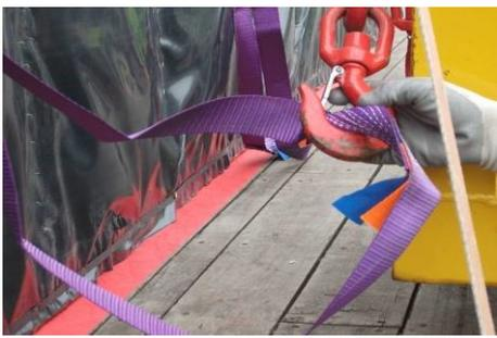
5. The crane will then take up the slack of the lift, and under instruction from the site responsible person the driver will release the transport straps on the side being unloaded.
