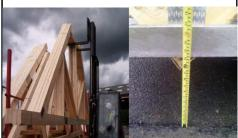
4. While the side loader supports the trusses the loader must tie back the truss pack to the centre bars or previous pack using minimum 6mm 3 core polypropylene blue rope (min 450kg
