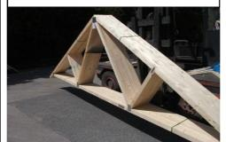
3. Suitable trailer must be selected with trusses loaded against centre bar or previous pack (ensuring that wherever possible it is the centre bars). Ensure all trusses are tightly packed and any inverted are a minimum 200mm from ground level.
