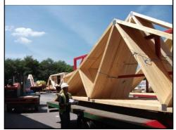
9. It is the drivers responsibility to inspect the load ensuring that it is safe for transportation. The driver will fit transportation straps to each side of the load
