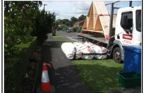
4. Pasquill will supply truss packs secured to the trailer with blue 3 core rope. You shall familiarise yourself with which rope attaches which pack to the centre bars.
