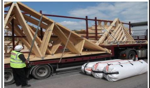
7. The driver will then cut the appropriate blue rope and banding to release the pack. The driver will safely mount the vehicle and release some of the tension on the small strap ensuring it is not completely removed.
