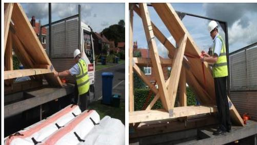
6. Once the load stability has been checked the driver will release the transportation straps from ground level ensuring the opposite side of the load is secure.
