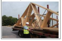
7. The driver will cut the individual rope attaching the pack to the bars. This must be carried out from a safe position using a closed blade pruning staff.
