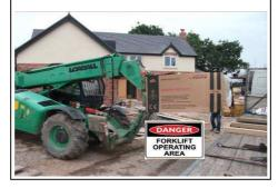
6. **NEVER** stand between the forklift and trailer, do not allow others to enter this danger area. **NEVER** stand on or under the forks. Ensure the danger area remains clear at all times.
