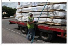
5. The forklift truck operator can now remove the packs and any palletised material from the vehicle. Ensure no one is within the danger area.
