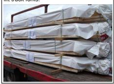
4. On instruction from the site responsible person the driver will release the transport straps on the side being unloaded ensuring no one is within the danger area as shown in the pictures.
