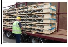
5. The forklift truck operator can now remove the beams and any palletised material from the vehicle. Ensure no one is within the danger area.
