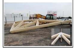
9. Once lowered the forklift will remove the forks and re-invert the truss pack at the apex. Once fully supported the truss pack can then be moved to its location.
