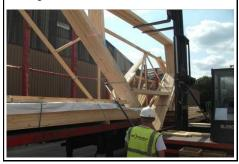
8. The forklift will then remove the truss pack from the trailer, position the apex of the pack onto the floor and reverse back slowly lowering the boom. Bearers can be used to support the underside of the pack
