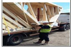
5. The operator must position the forklift in an appropriate area to ensure the trusses are lifted safely. The forklift will take the weight of the trusses on the forks. Ensure no one is within the danger area.
