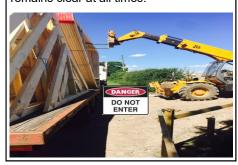
7. Once the pack is supported the driver will cut the individual rope attaching the pack to the bars. This must be carried out from a safe position using the drivers cutting tool.
