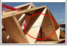
4. the On instruction from site responsible person the driver will release the transport straps on the side being unloaded ensuring no one is within the danger area as shown in the pics 5-8.
