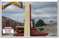
8. The forklift truck operator must lift the trusses from the trailer and then move the trusses to a safe and / or off-load storage area.
