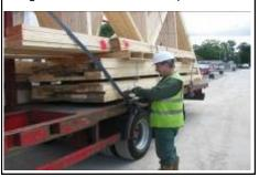
7. The driver will cut the individual rope attaching the pack to the bars. This must be carried out from a safe position using the drivers cutting tool.
