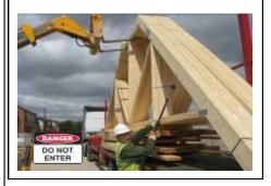
5. The operator must position the forklift in an appropriate area to ensure the trusses are lifted safely. The forklift will take the weight of the trusses on the forks. Ensure no one is within the danger area.
